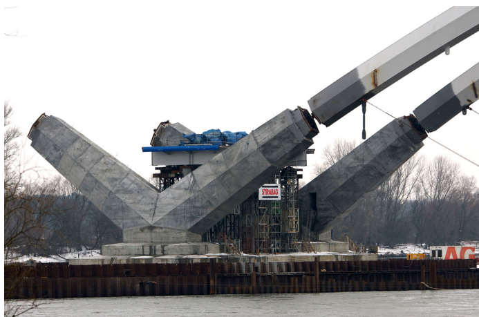
Fig. 4. Central pier - installation load.
