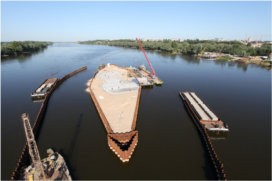
Fig. 6. The island after the completion of piling works.
